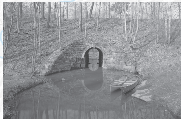
Ross Creek Stone Culvert
