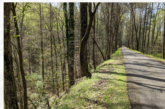
Brock's Gap: Tall fill bridging the valley between Shades and Pine Mountains
