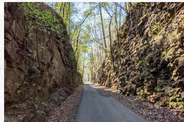
Cut through Pine Mountain at Brock's Gap
