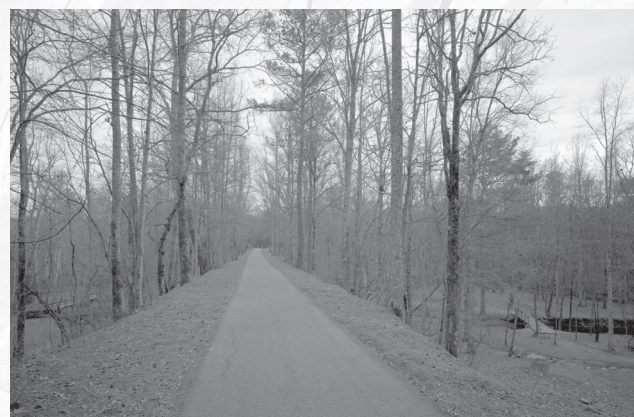
South & North Alabama RR embankment above Ross Creek
